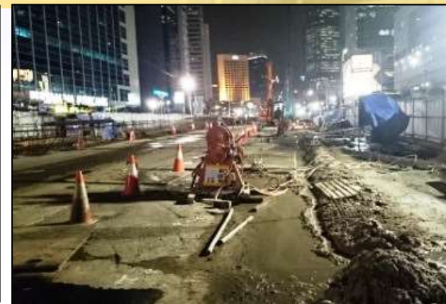
Dukuh Atas Station: Soil Improvement
