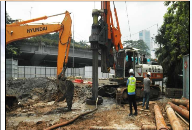
JI. TB Simatupang: Point Square LP 7 and LP 8 Permanent Pile
