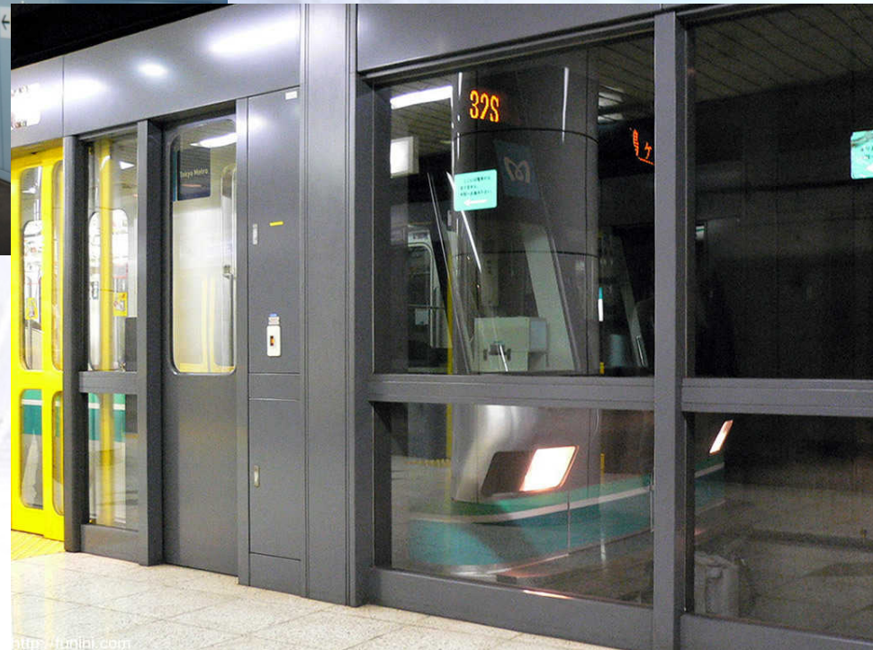
Underground Station (Full-height Type)
