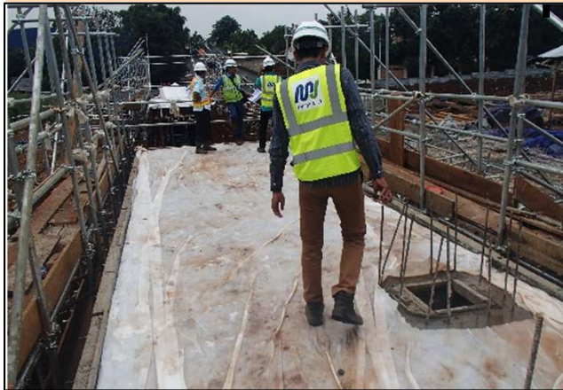
LBBT: Box Culvert Section B&D pouring concrete finished
