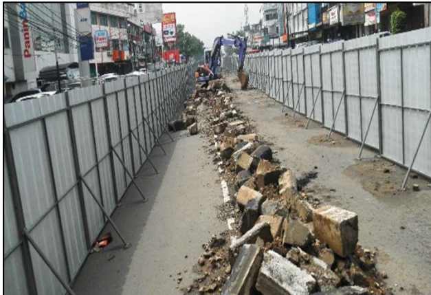
Jl. Fatmawati, FP-16 to FP-30 Barricade was installed
