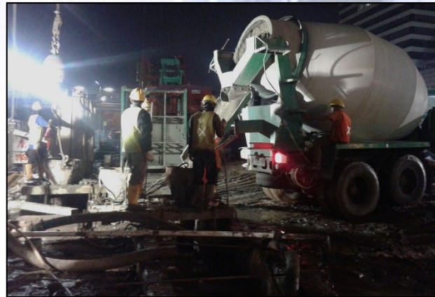
Istora Station : Pouring Concrete D-wall P76
