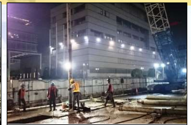
Bunderan HI Station : Tremie Pipe Installation for D-Wall34
