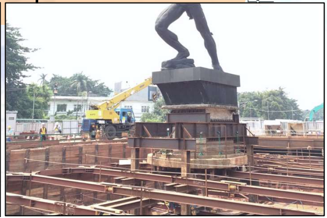
Transition Area: Soil Excavation layer 2 at zone 2
