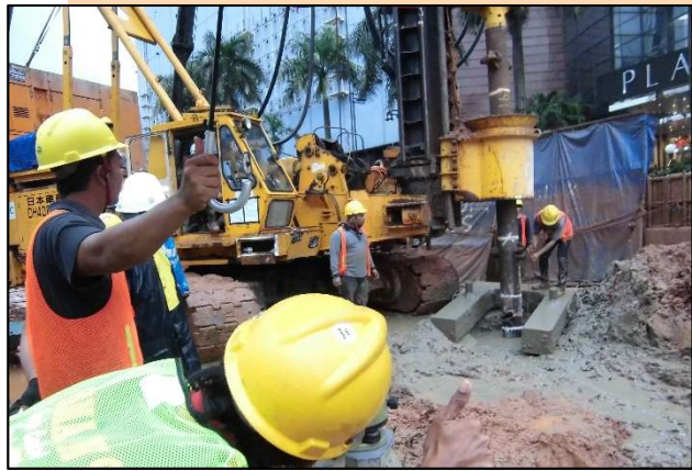
Blok M (Center Median) : Pilling MS 11 C No Pile 4
